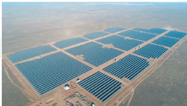
Maloderbetovskaya Solar Facility, Kalmyk Republic
