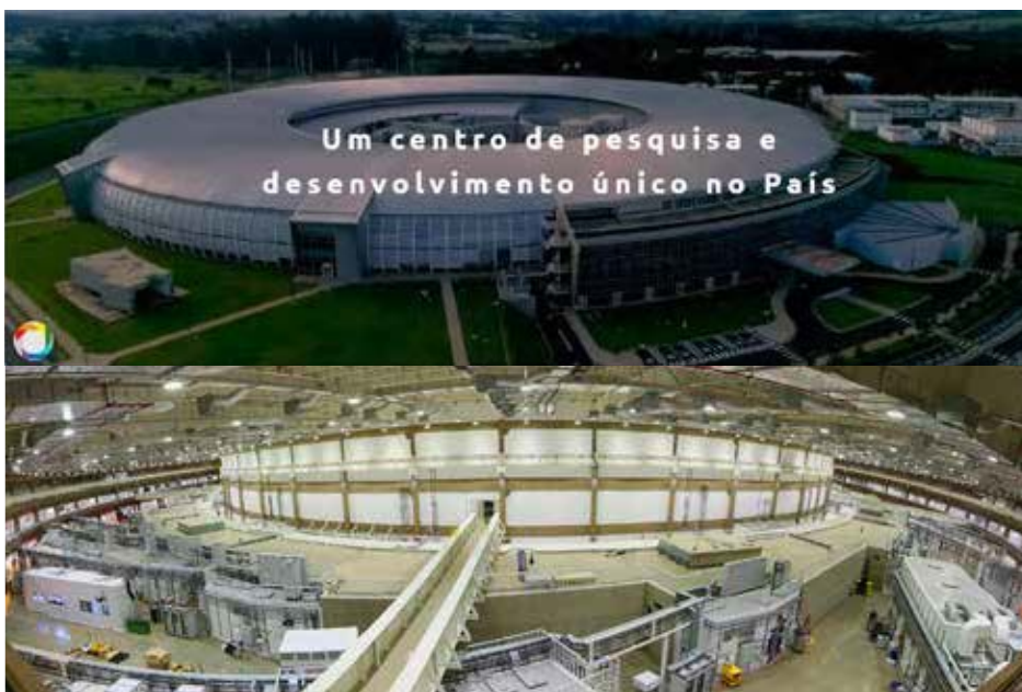
Figure 2.10 – Sirius: the Brazilian synchrotron light source (external and internal views)
